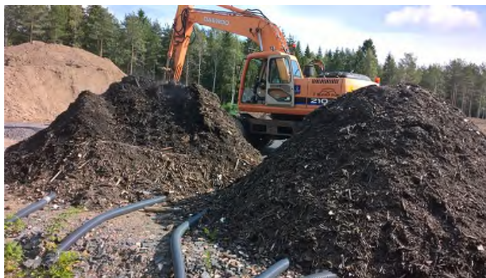
Figure 26. Composting test heaps were constructed in July 2017.
